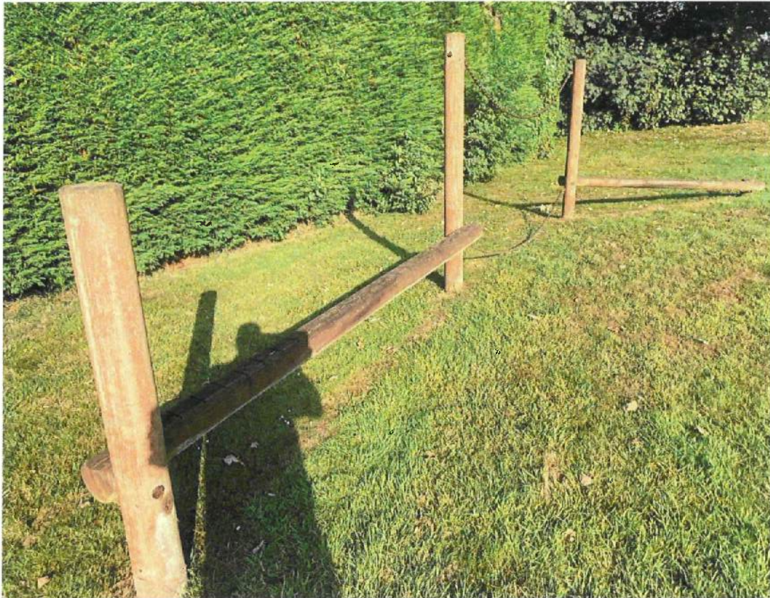
Strimmer damage, splits and rot on balance beams.
