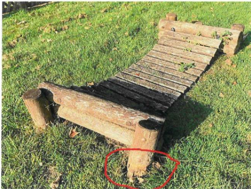
Timber bridge support leg has failed requires replacing
